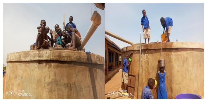
The conduits connecting the tanks and the roof through the gutters is disconnected to that when the first rains sets in, the dust and dirt that was gathered on the roofs and gutters are washed away instead of getting into the tanks. The conduits are reconnected to allow clean water to be harvested after a few rains.
