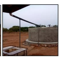
The gutters are connected to the tank awaiting the first rains to wash and clean the inside and to ensure that the tank would be able hold the water with no cracks.
